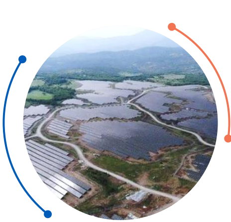
Borusan EnBW GES* 94 MWp | Türkiye | Arazi GES
