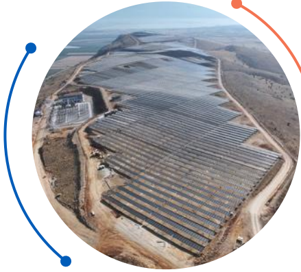
Deski GES 90 MWp | Türkiye | Arazi GES
