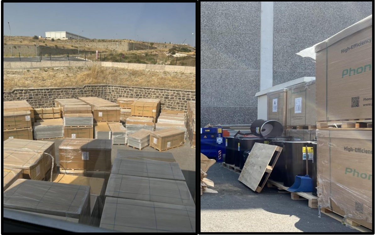
Figure 3-22. Panel Stacking (left) and Packaging Waste Storage (right)
